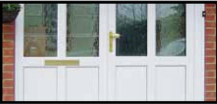
It is possible to form a 'crucifix' joint above and below the midrail by combining a vertical mullion and the horizontal midrail.
